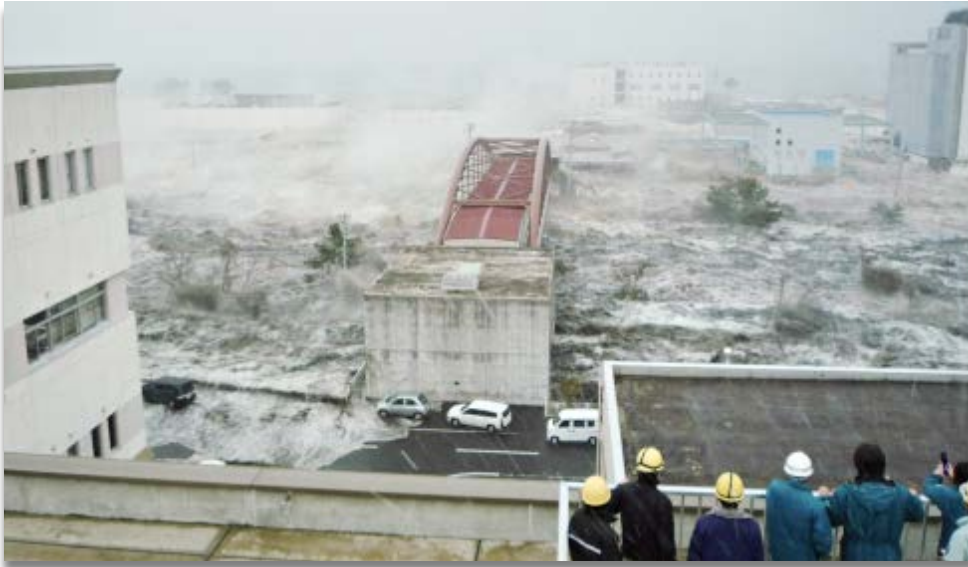
Figure 3: Flooding and evacuation of Minami-Gamo Wastewater Treatment Plant after the tsunami on March 11, 2011 (Sendai City Construction Bureau 2013).
